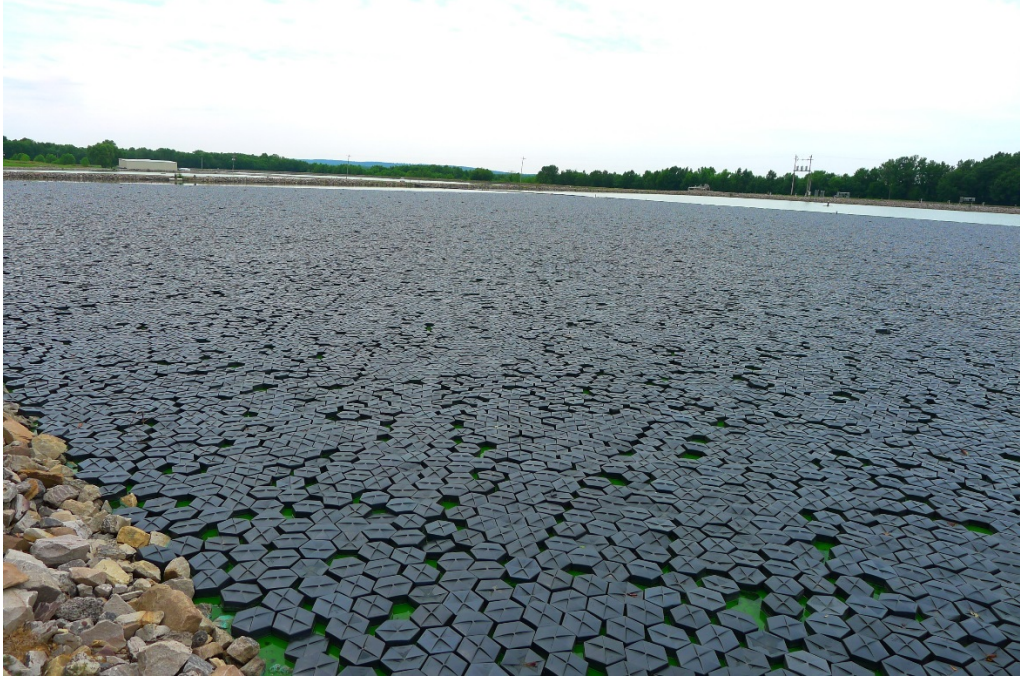
Photo 1 Hexprotect Floating Cover Tiles
