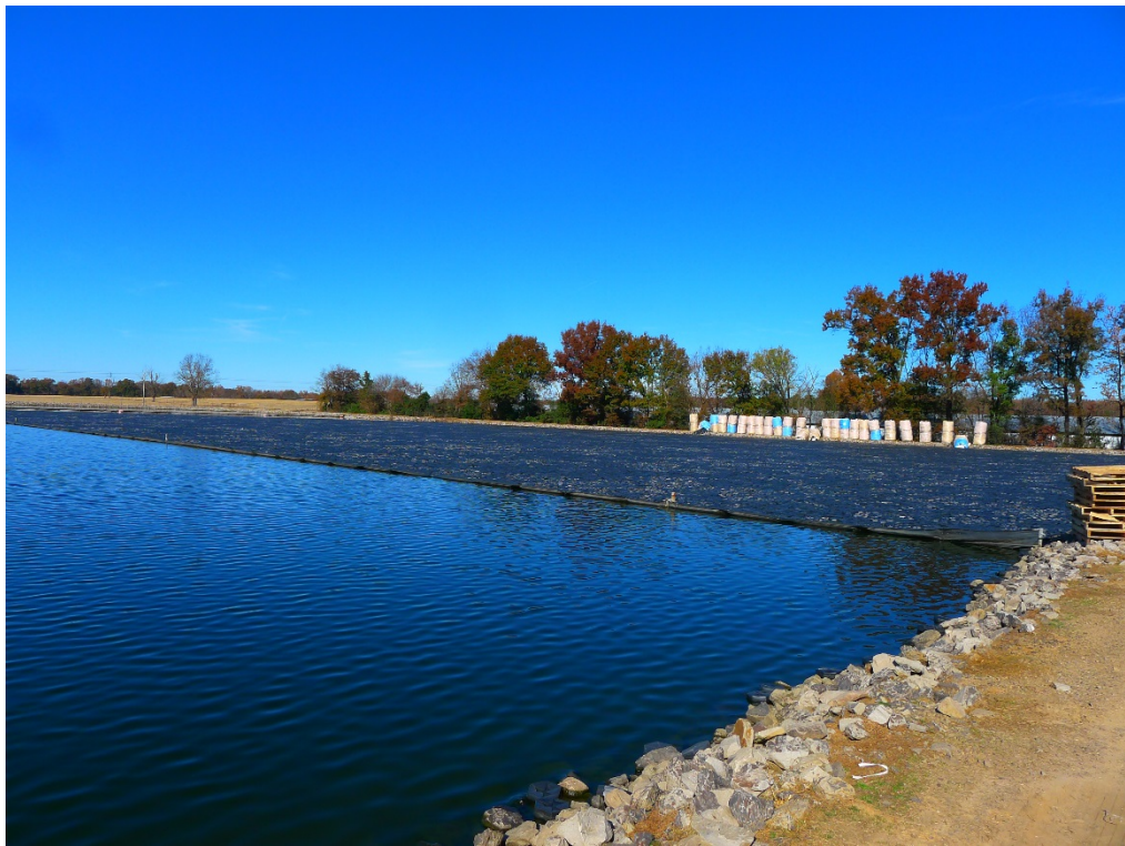
Photo 2 Tiles Contained in Lagoon 2
