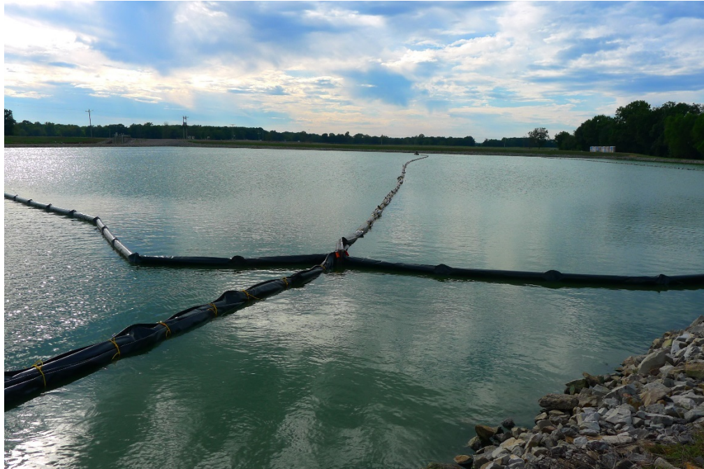
Photo 3 Installing the Assembled Baffles and Booms
