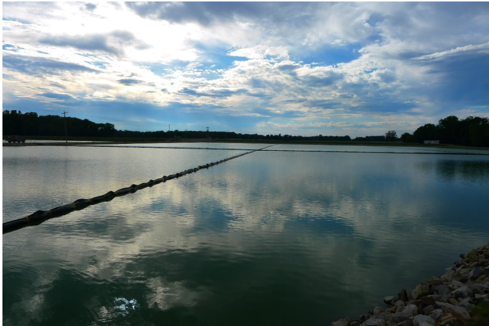
Photo 4 Baffles and Booms in Place
