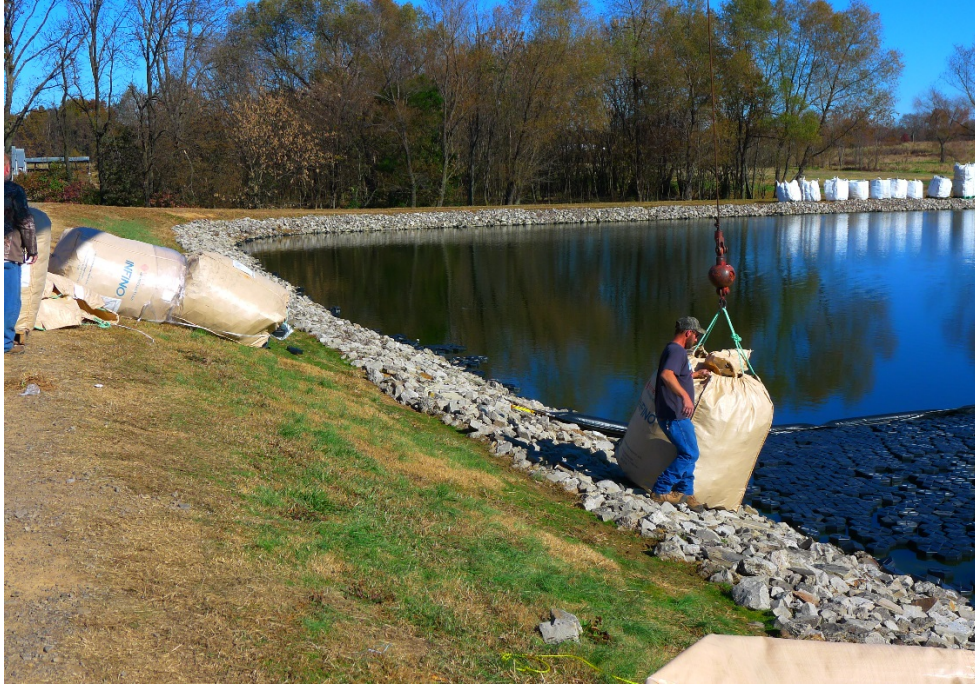
Photo 7 Installing Hexprotect Tiles
