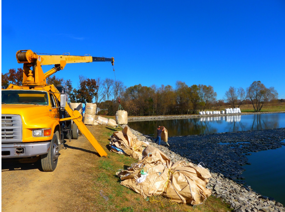
Photo 5 Installing Hexprotect Tiles in Lagoon 3
