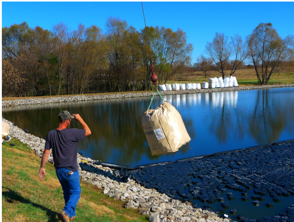
Photo 6 Installing Hexprotect Tiles
